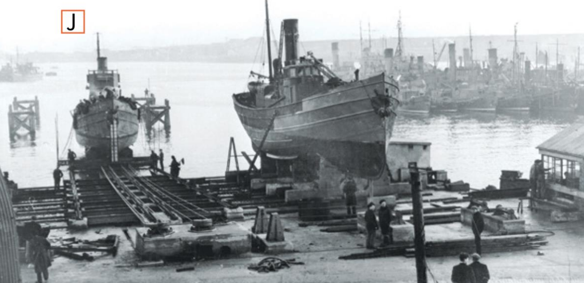
J. Upgraded in 1944, the drifter slipway allowed quick repair of up to 3 boats at a time. See point No.16.
