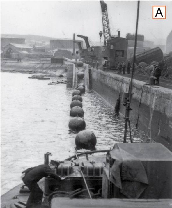
A. An anti-submarine boom net being launched from the net runway alongside Lyness Wharf.
