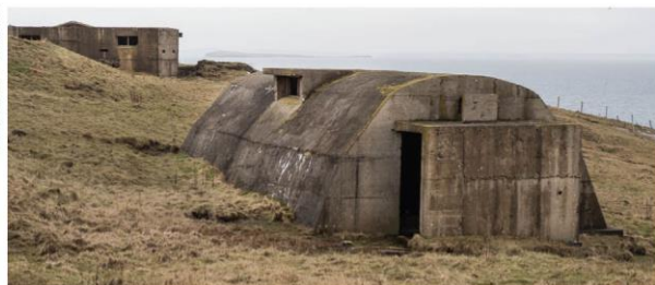
WW2 engine house in a reinforced Nissen hut, Hoxa Battery, 2022
