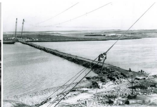
August 1943. The barrier nearing completion as seen from Lamb Holm. Note the aerial ropeways.
